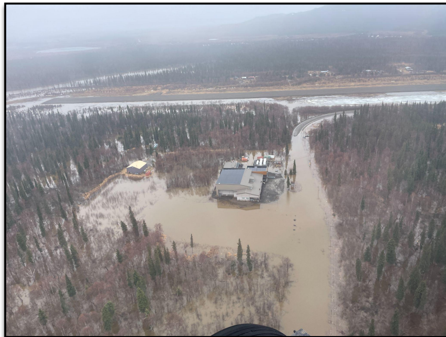
Aerial view of flooding around airport runway, with water surrounding homes and structures and flooding of the roads between Upper and Lower Kalskag - May 17th.
