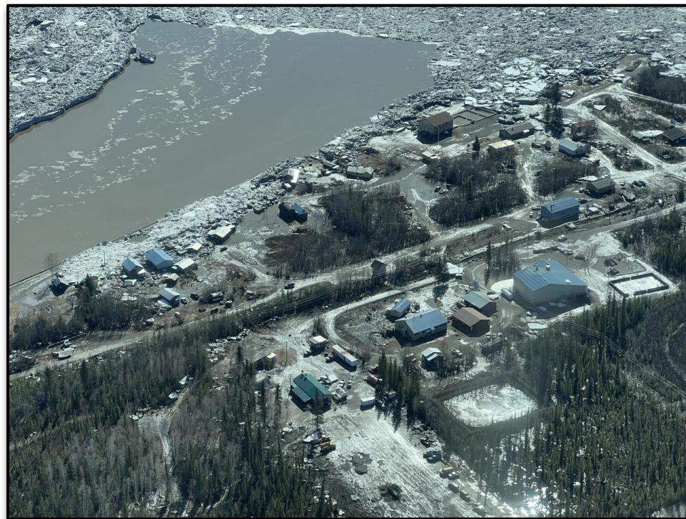
Stranded ice and floodwaters in Circle with residential structures damaged shifted off foundations - May 14th.
