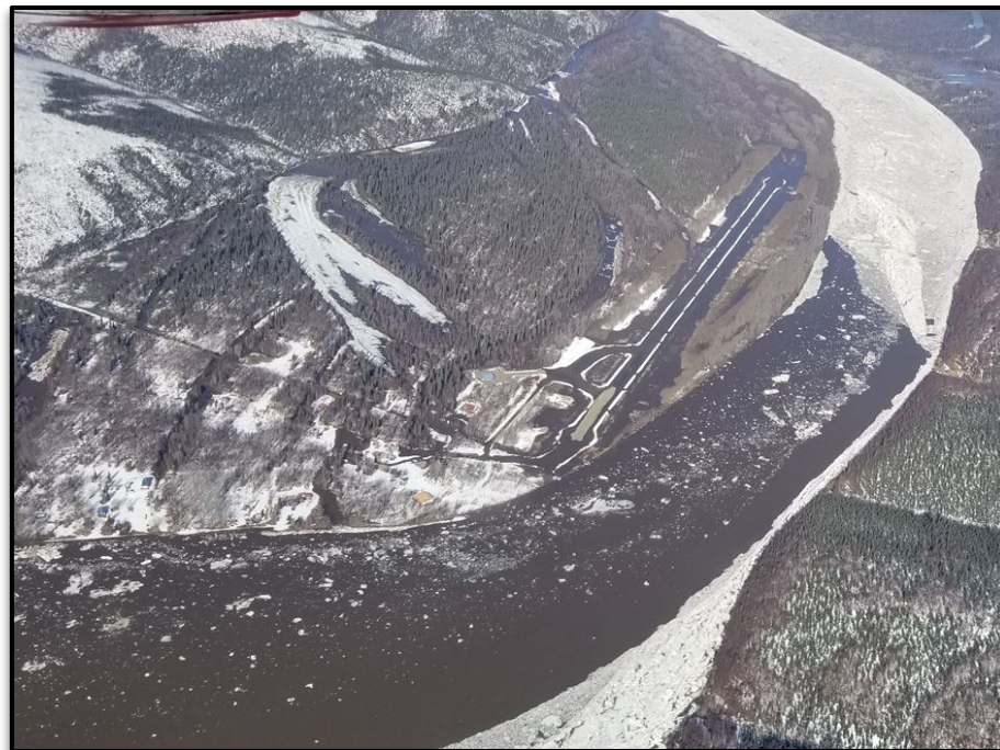
Aerial view of Red Devil showing extensive flooding to the runway on May 13th.
