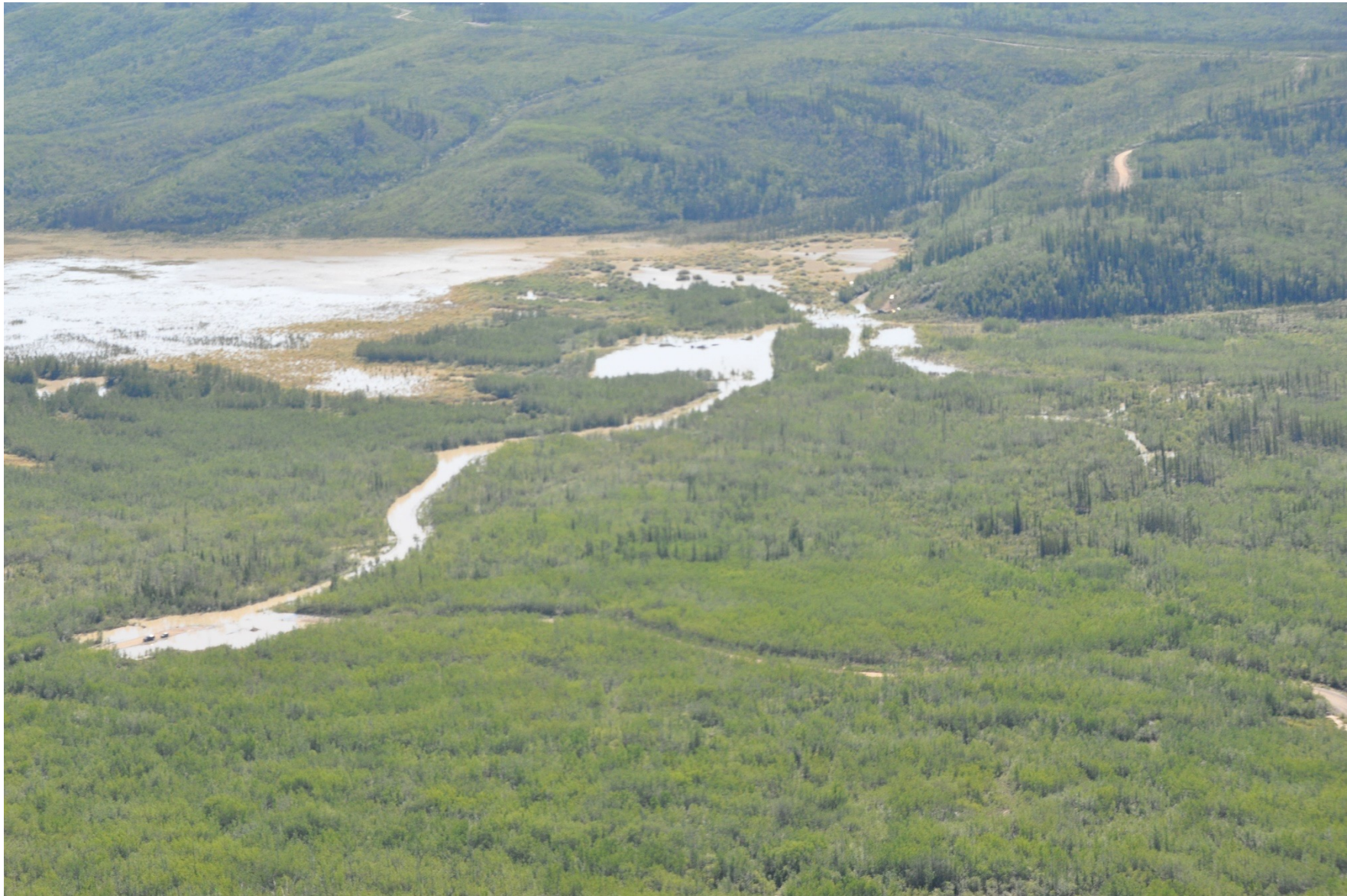
Civil Air Patrol Flight, August 5 th Looking Southeast at the Flooded Portion of the Road
