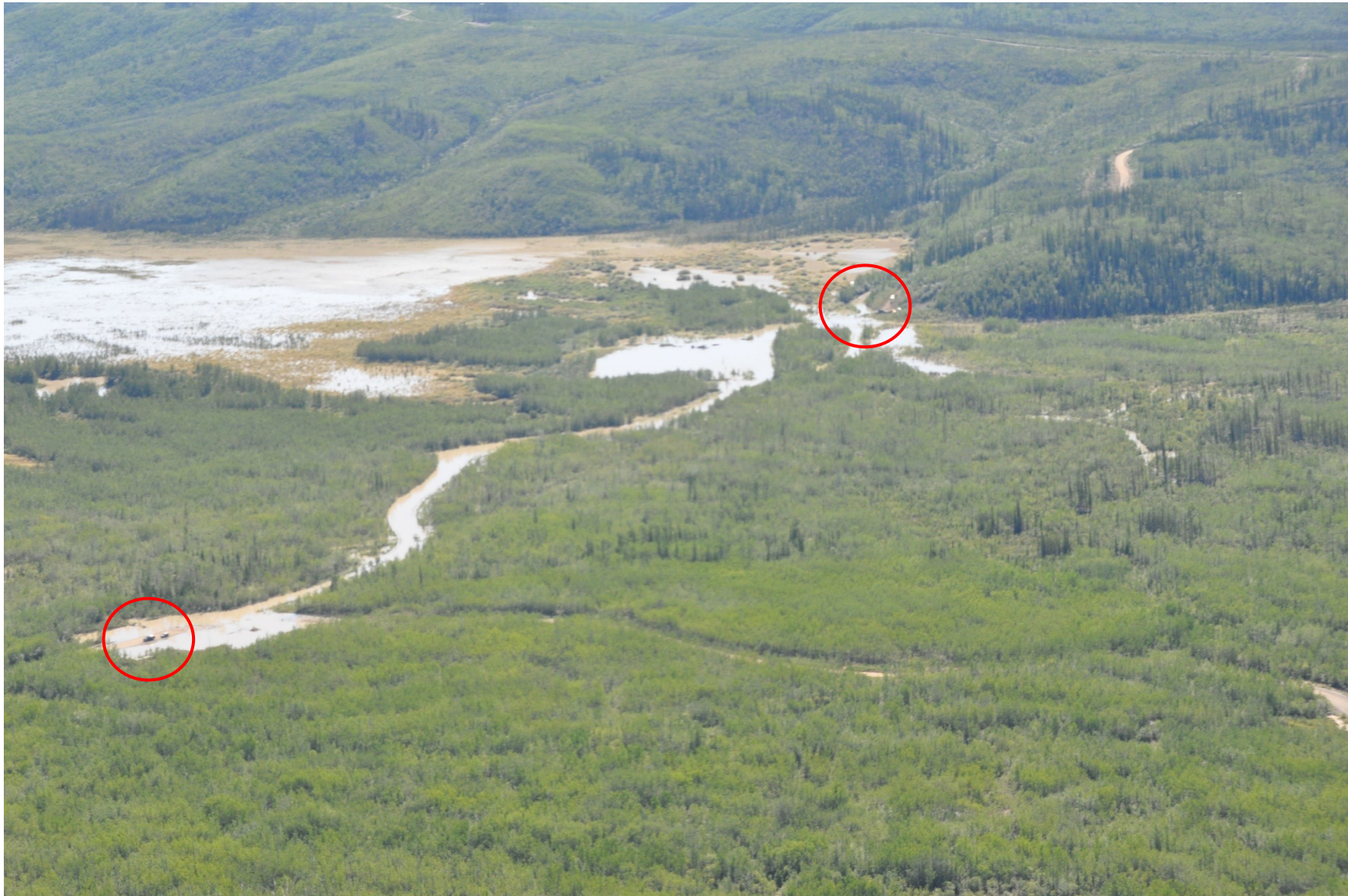
Civil Air Patrol Flight, August 5 th Looking Southeast at the Flooded Portion of the Road
