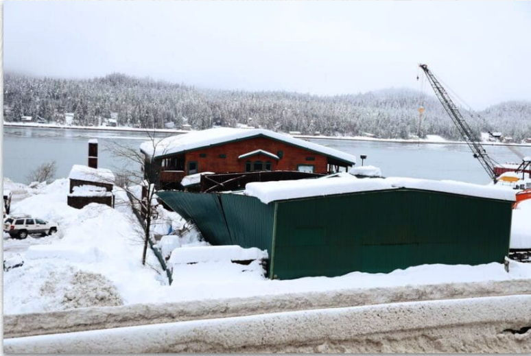
Roof collapse in Juneau
