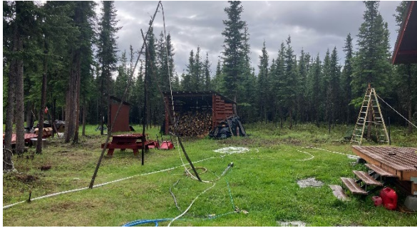
Structure protection using sprinklers on recreational cabin threatened by the McDonald Fire in 2024.
