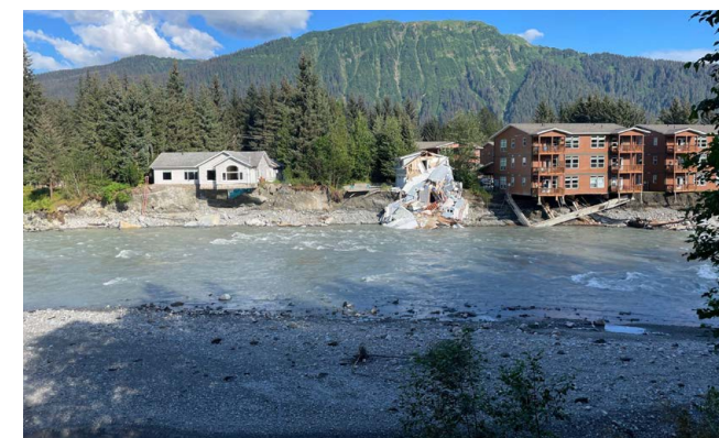
August 2023 Mendenhall River looking at a house that fell into the river and another damaged house. Photo by Juneau NWS.
